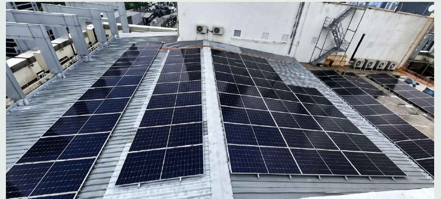
A rooftop solar panel system was installed at Kenanga Tower to increase the share of electricity sourced from renewable energy, supporting our efforts to decarbonise Scope 2 emissions under the Decarbonisation Roadmap.
